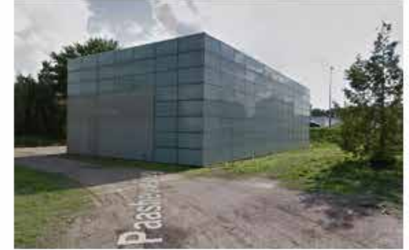
Warmte Overdracht Station Paasheuvel 4, Bullewijk Cepezed
