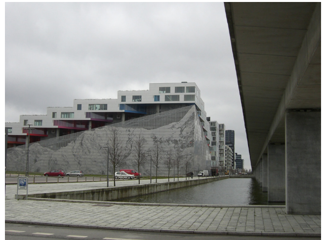
img. 55: Residential building next to metro line
