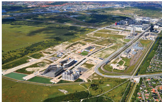
img. 50: Arial picture starting point of execution and metro line
