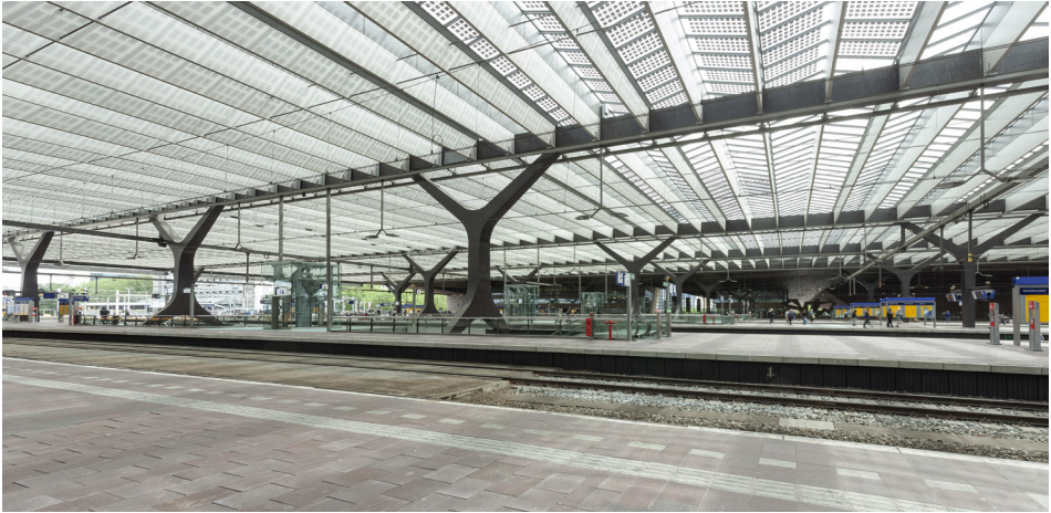
Figure 7.1 Original photo of the built environment of Rotterdam Central
