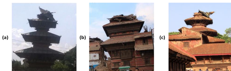
Figure 2: Different cases of collapse of the top part of the Nepalese temples during the Gorkha earthquake that hit Nepal in 2015, (a) (Endo and Hanazato, 2019), (b) and (c) (Shrestha, 2015).
