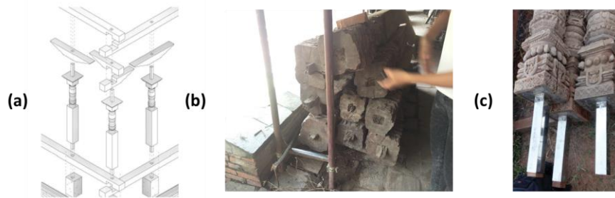
Figure 1: (a) Detail of the connection of the wooden pillars with the rest structural elements (Arce et al. , 2018), (b) typical failure of the vertical timber elements supporting the peripheral walls, and (c) strengthening of timber pins with stainless steel warping (Arce et al. , 2018).
